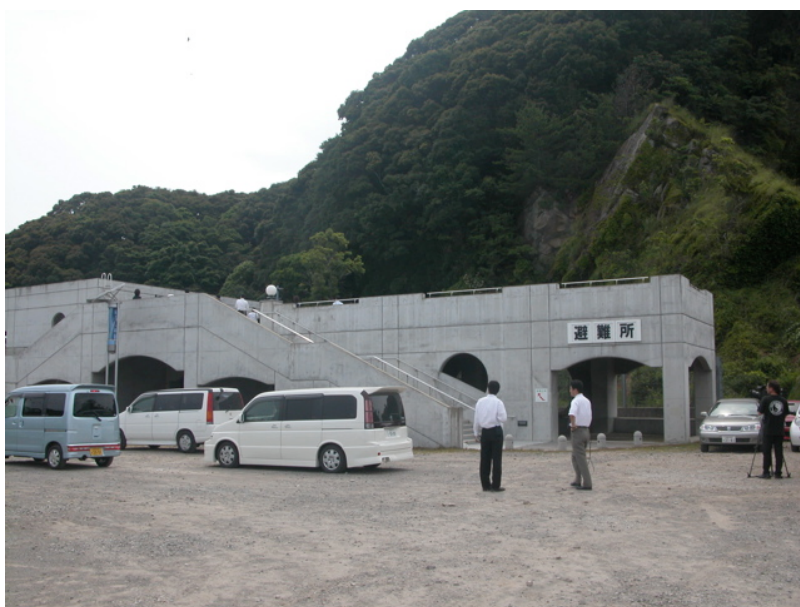
Fig.1 Tsunami shelter, Sange district
